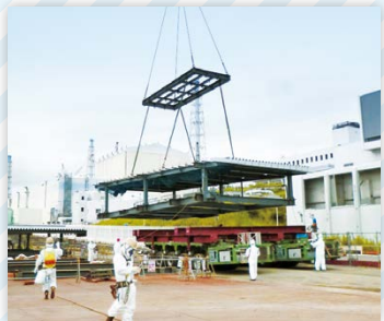
Power plant maintenance
