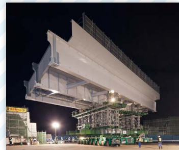
Bridge erection and dismantling
