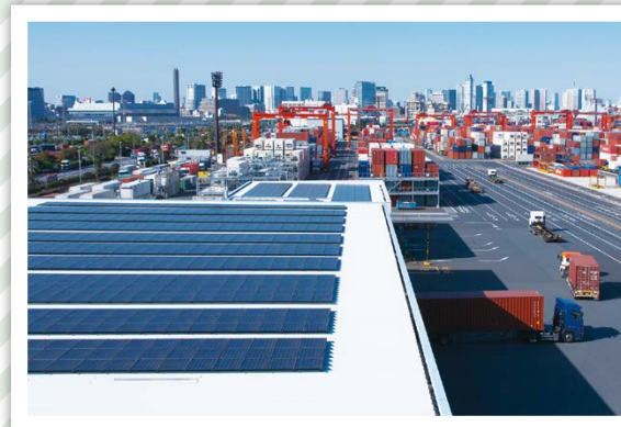
Our Tokyo International Container Terminal is the first port facility in Japan to operation solar power generation.
