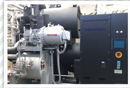
As part of our commitment to prevent global warming, we switch the cooling equipment of cold warehouse from the equipment that uses freon gas, which uses a high greenhouse effect, to the equipment that uses natural refrigerant (non-freon freezer).
