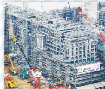
Plant construction/maintenance (overseas)
